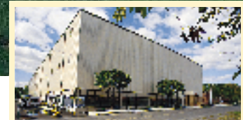
Cable and Wire Plant
